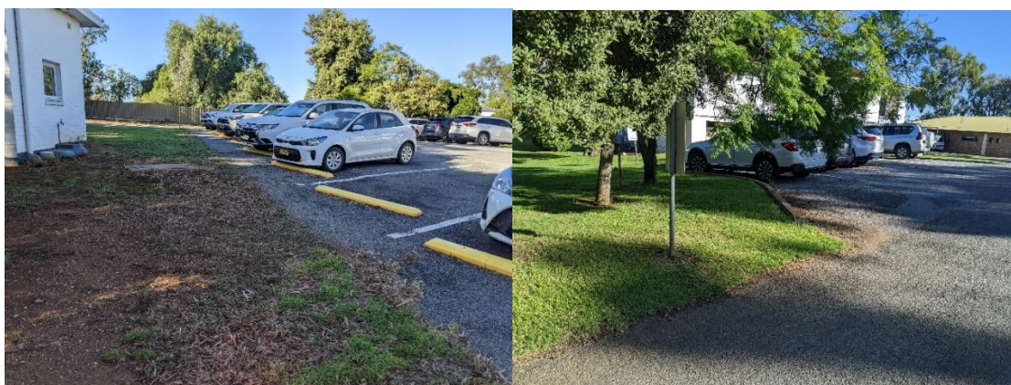
Asphalt/Gravel carpark in the North-East (L-Eastern End, R-Western End)
