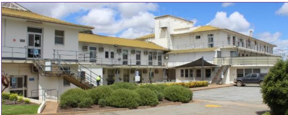
Existing Temora Hospital (Eastern Elevation, viewing North)
